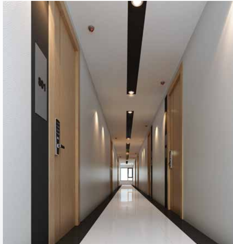
KEY CARD, FIRE ALARM, DIGITAL DOOR LOCK
